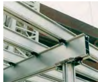
Headplate to beam fixing
