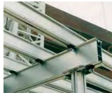
Headplate to beam fixing
